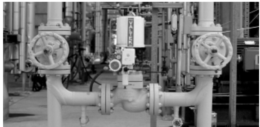
This eight-inch, back-pressure control valve operates in a liquid hydrocarbon plant with a 580 psi / 40 Bar upstream pressure.
