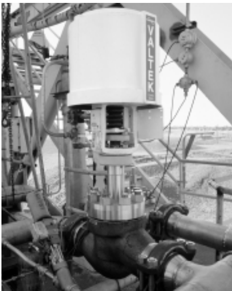
This cryogenic Mark One is used for aerospace testing as an LO 2 vent valve.
