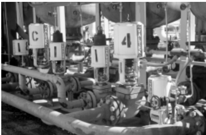
This cryogenic Mark One is used for aerospace testing as an LO 2 vent valve.
